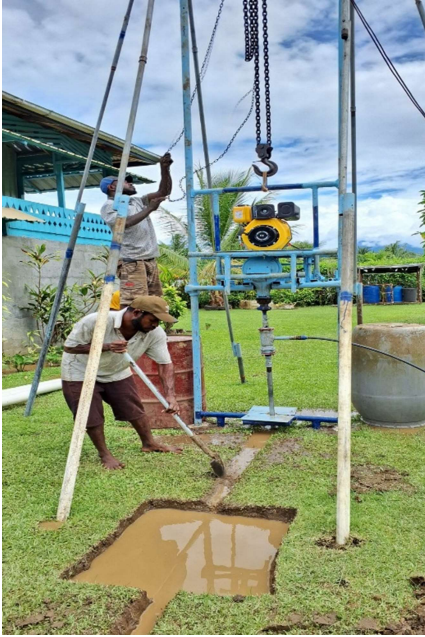
Borewater drilling
