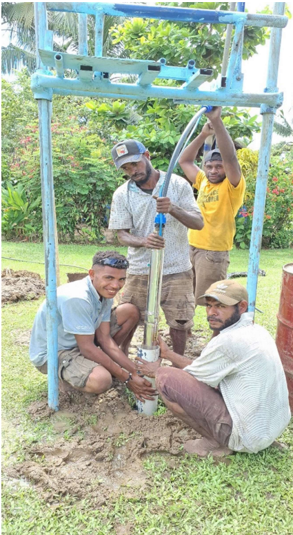
Installing deep well water pump
