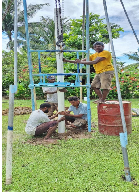
Installing borehole casing
