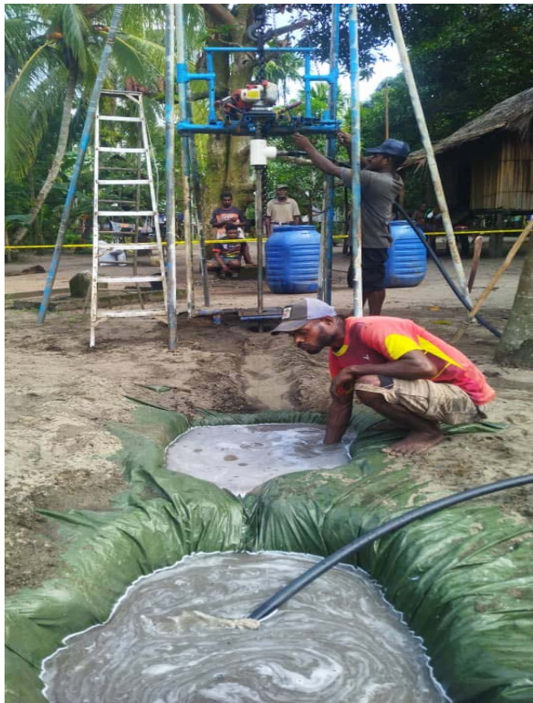
Water drilling mud setup
