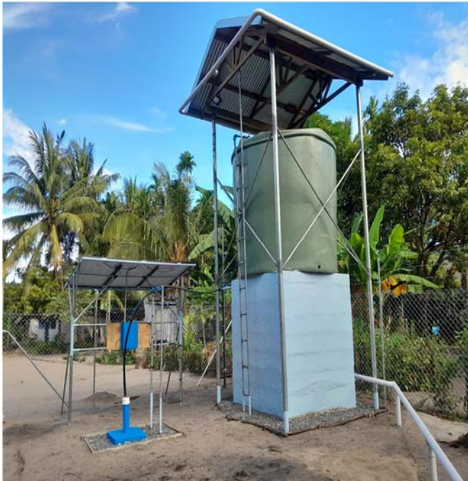
Completed sustainable smart water system
