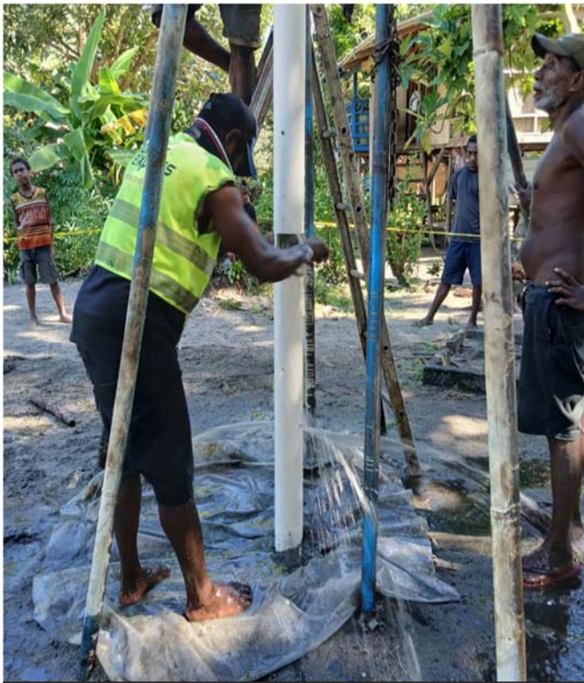
Inserting borehole pressure pipe casing
