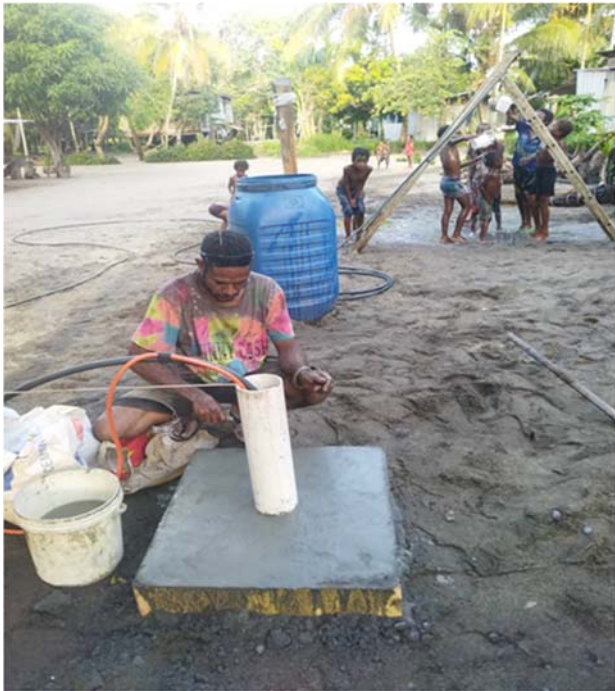
Borehole sealing and monitoring
